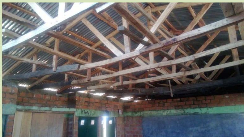
Figure 1 A cross-section of the renovated roof
